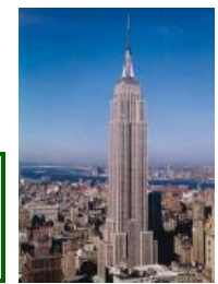
Empire State Bldg
